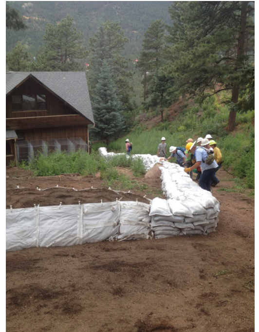
Sandbag wall with a sharp turn/angle. A large rock and a drop off prevented a gentler turn.
